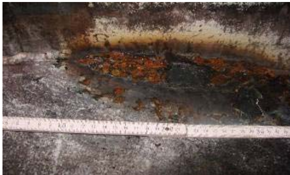
Hr.Ms. "De Ruyter" (LCF 3). Sewage storage tank: Corrosion on tank bottom
