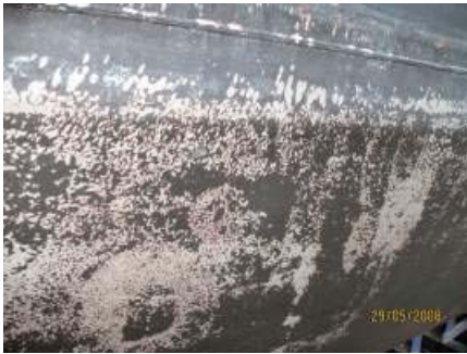
Paint system failure
